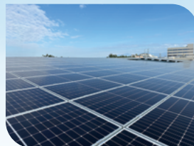
▲ Installation of solar power systems in the plant area
